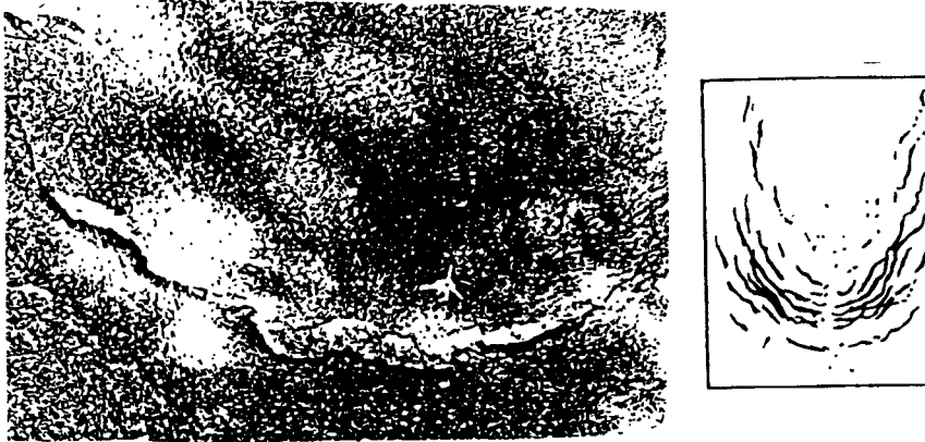
Gambar 8.8. Retak selip ( slippage cracks )
