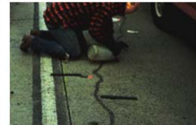
4. Pouring epoxy into drilled holes (Injecting epoxy is preferable for large quantities)
