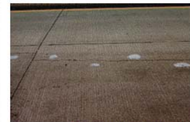
6. Completed cross-stitching on longitudinal joint.
