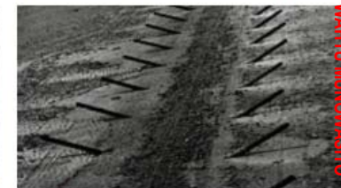
5. Inserting bars into prepared holes containing epoxy. (Note: The bars shown here are in position but not fully inserted.)
