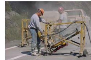
1. Drilling hole for tie bar along longitudinal crack using frame-mounted drill rigs.
