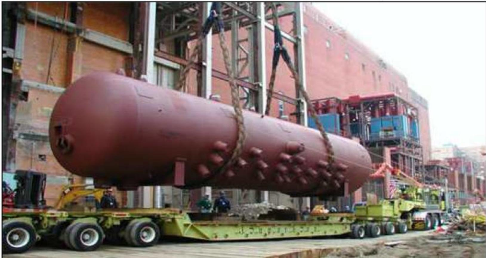
**Gambar *Drum Boiler*.**
