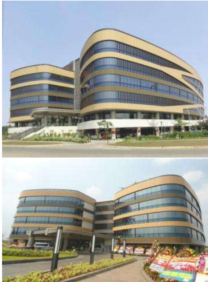
Green Office Park 6 - BSD IGU: 8mm T-CS 140 +AS12 +Panasap Dark Blue 6mm
