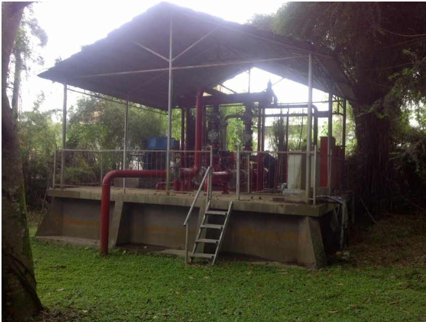
Rumah pompa terbuka. Lift suction. Main pump listrik merk Torishima – non listed
