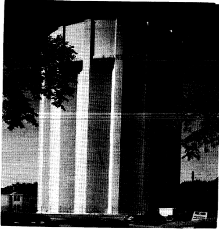
Fig. 14.26. Municipal water tank of Topeka, Kansas. A vertical cylinder on the inside, this water tower on the outside seems to consist of vertically bisected cylinders with the concave outward.
