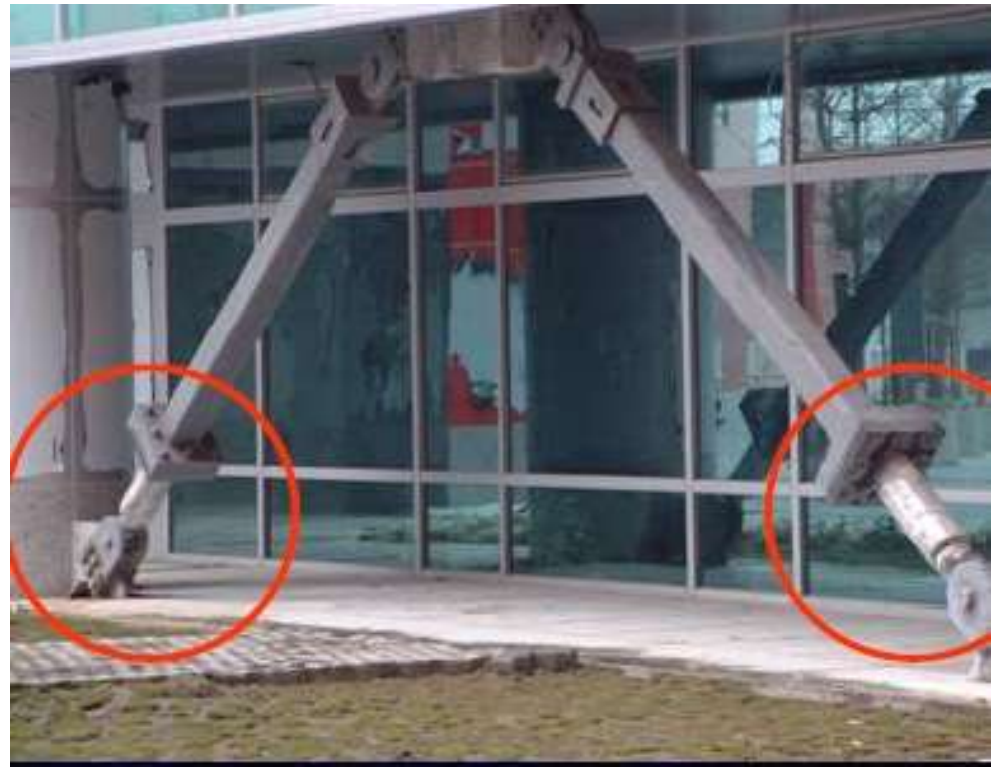
Energy dissipation bracing type
