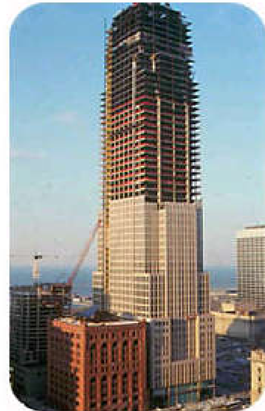
High-strength silica fume concrete was used to stiffen the Key Bank Tower in Cleveland, Ohio.
