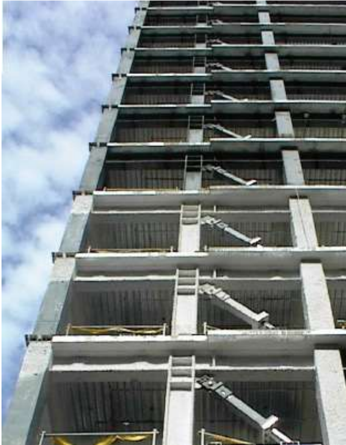
Energy dissipation bracing type
