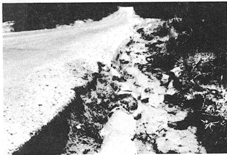
Gambar 2.20. Lane/Shoulder Drop Off
